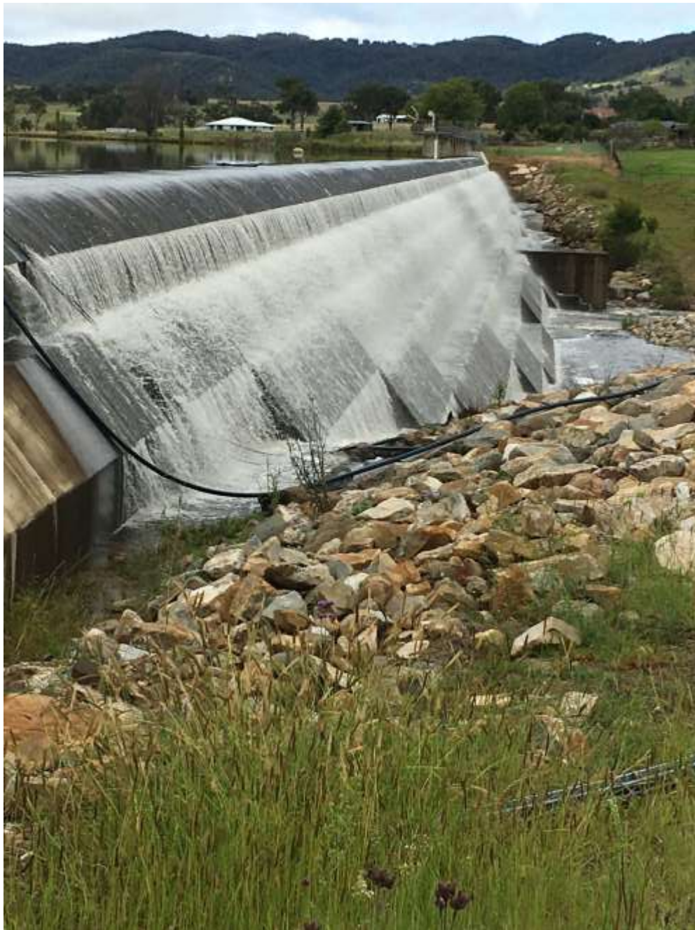
Figure 1: View of Dam Wall March 2022
