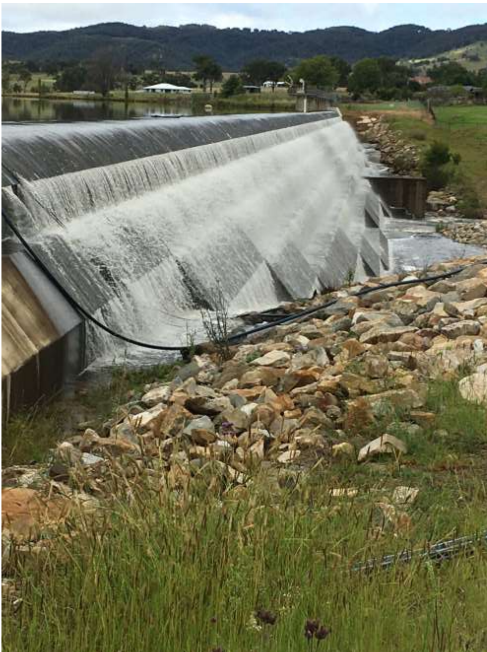
Figure 1: View of Dam Wall March 2022
