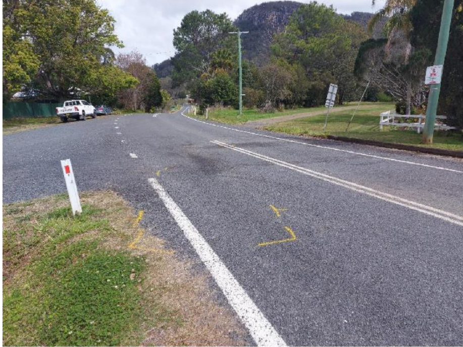
West bound view of accident site
