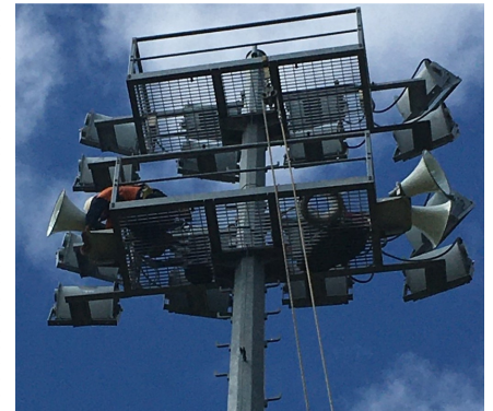
Installation of sirens for the upgraded Flood Warning System, Photographer G. Marchant, Manager Water and Waste
