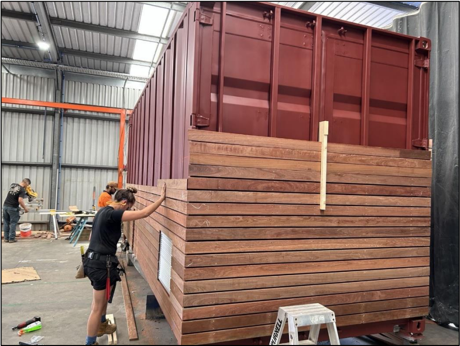
Image 3 - External cladding being fitted.
