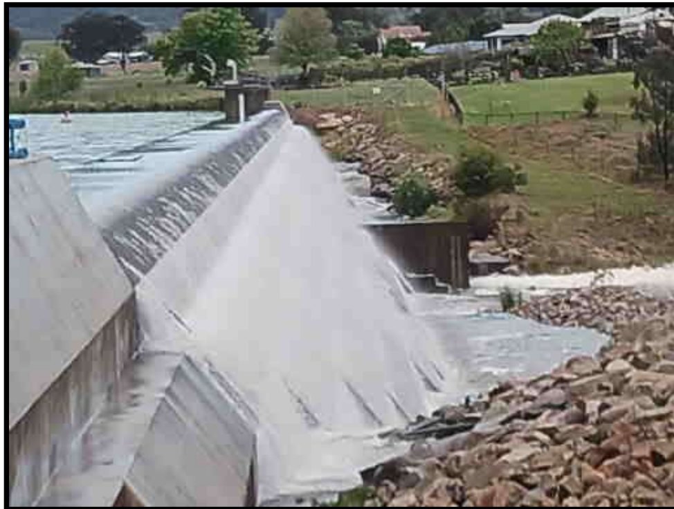
Figure 1: View of Dam Wall October 2022
