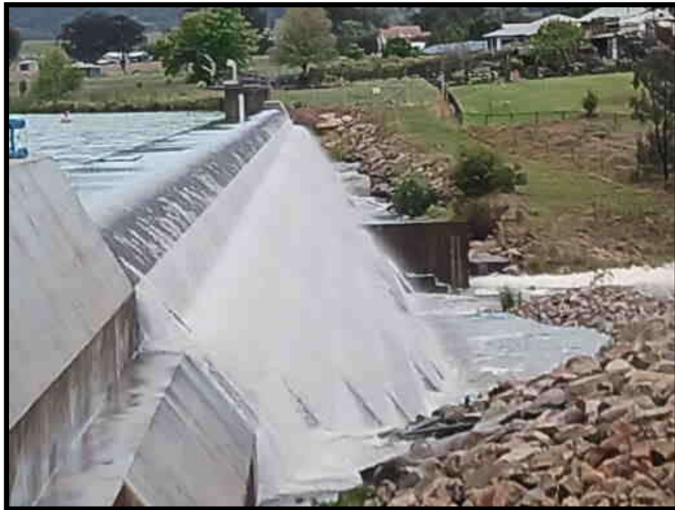
Figure 1: View of Dam Wall October 2022
