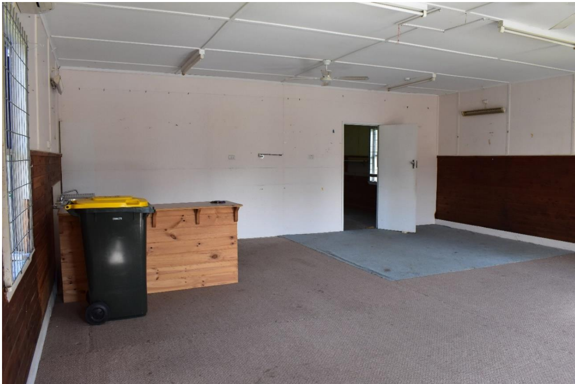
Figure 2.17 – Facing north-west across main hall area showing non-structural internal partition wall.
