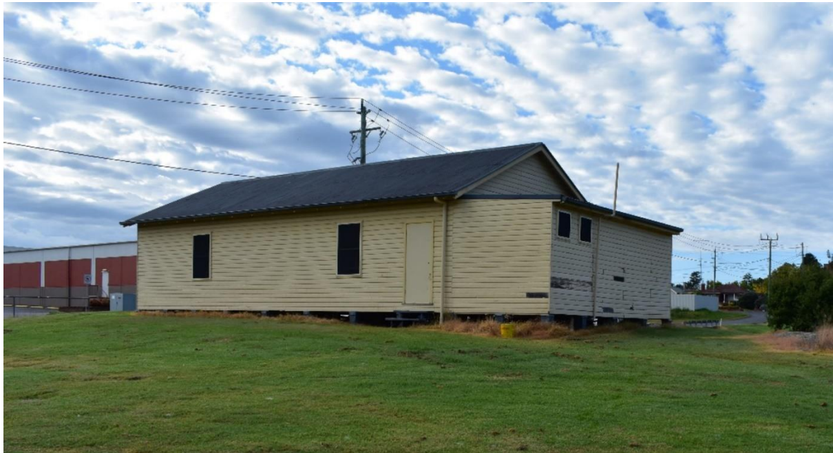
Figure 2.23 – External view of northern elevation showing the rear skillion addition for toilets and kitchen. The rear door may be a later modification.
