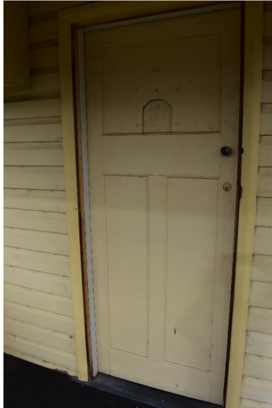
Figure 2.12 – Detail of solid timber entry door with RAOB peep-hole.
