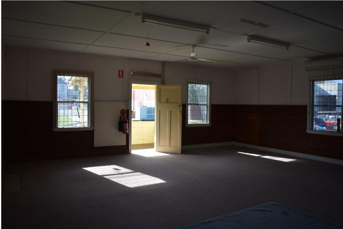
Figure 2.16 – Across main hall area to entry door showing internal wall and ceiling linings, likely to be fibre based sheeting with cover boards, typical of buildings prior to the 1970s. The timber lining on the lower walls is laminated sheeting popular in the 1980s and likely installed about the same time as the partition wall.
