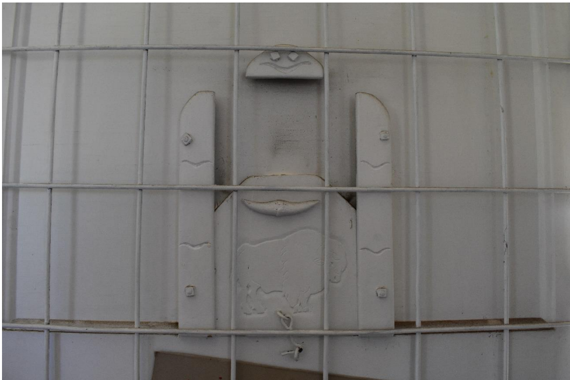
Figure 2.15 – Detailed view of internal peep hole installed by the RAOB with engraved Buffalo insignia. This element should be retained.
