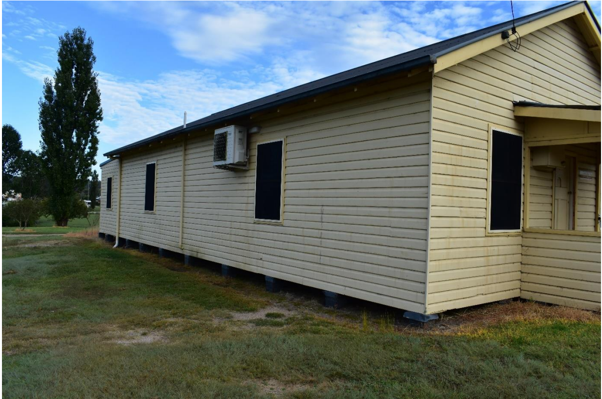
Figure 2.22 – External view of southern elevation showing brick piers.
