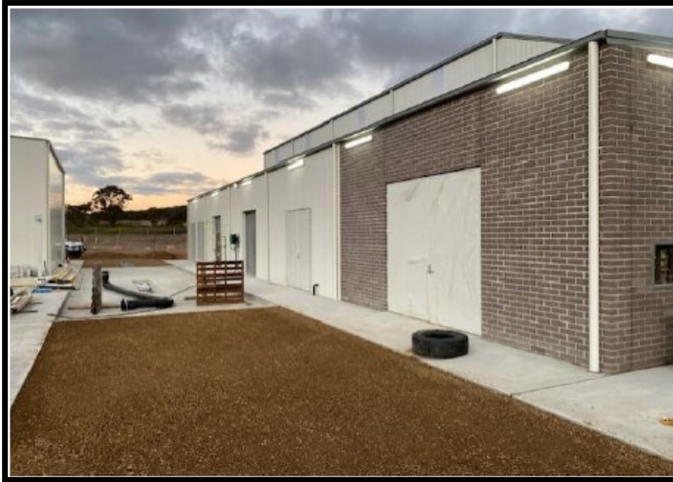
Tenterfield Water Plan security and lighting system.
