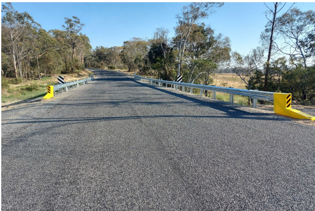
Mount Lindesay Road at Bookookoorara completed bitumen sealing of the road.
