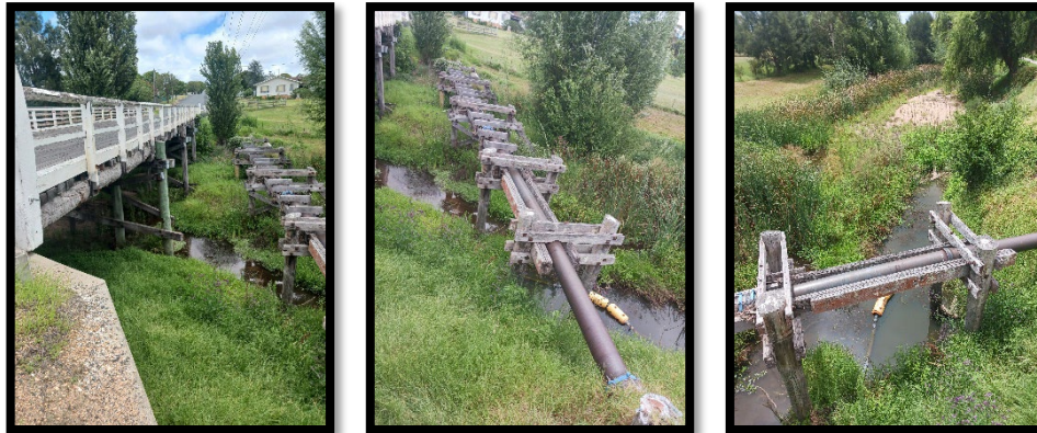
Figure 1, 2 & 3 Molesworth Street sewer aqueduct
