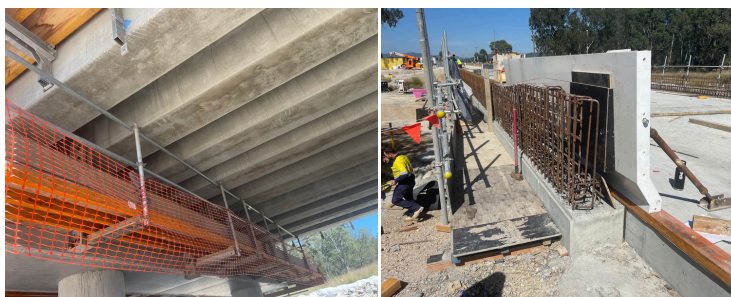
Dumaresq Bridge (Black Creek)
