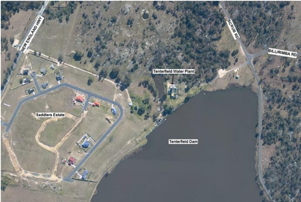
Figure 2 Tenterfield Water Supply Dam & Water Treatment Plant
