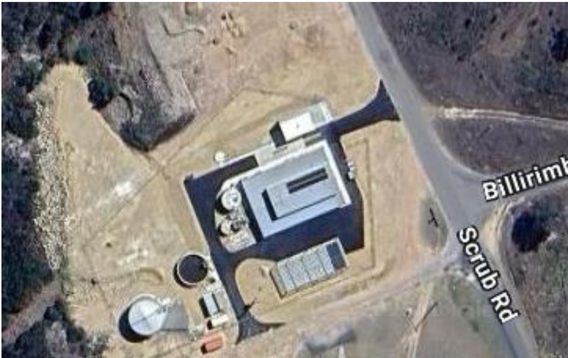
Figure 3 Tenterfield Water Treatment Plant
