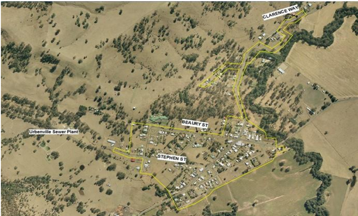
Figure 13 Urbenville & Sewerage Treatment Plant
