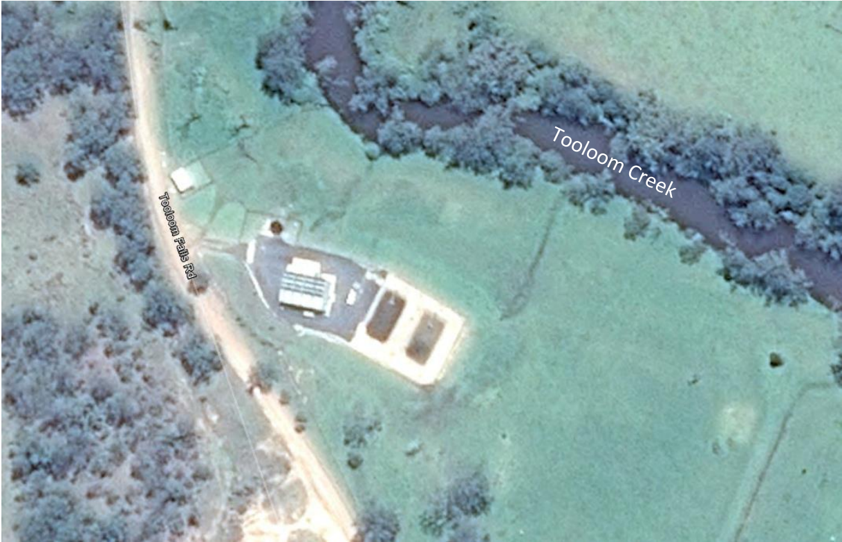
Figure 5 Urbenville Water Treatment Plant
