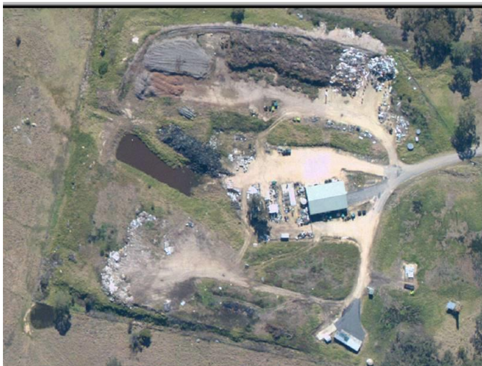
Figure 4-3 Tenterfield Waste Transfer Station
