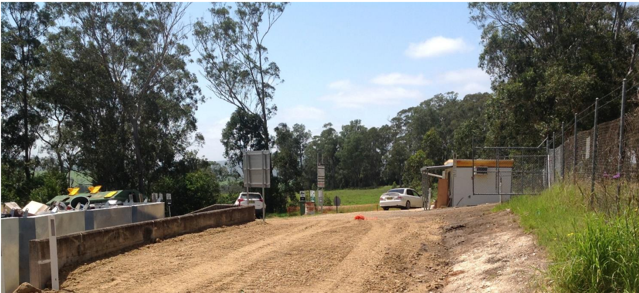
Figure 4-4 Urbenville Waste Transfer Station
