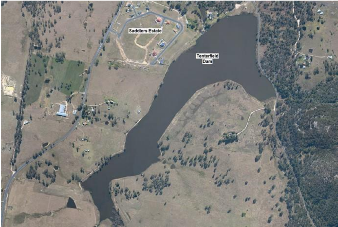
Figure 1 Tenterfield Water Supply Dam
