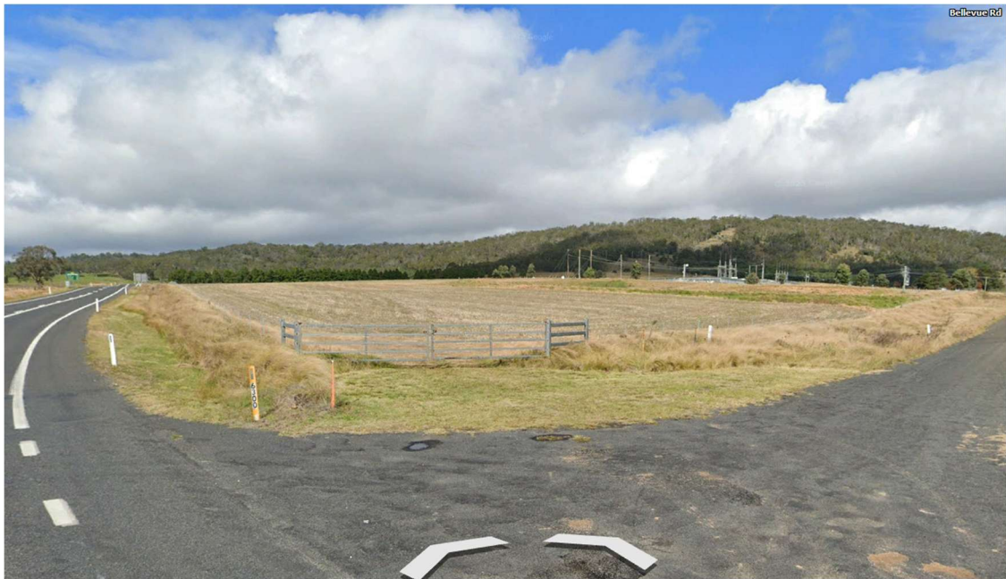
Intersection of Bellevue Road and Bruxner Highway to south-west of site Essential Energy Tenterfield 132kV substation visible in background
