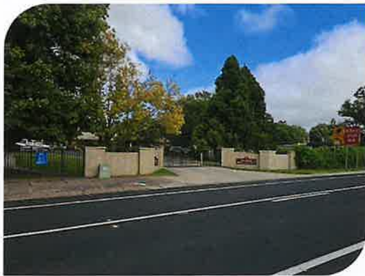
Figure 5 – Looking west from Rouse Street towards the Site Source: K+C, 3 February 2026
