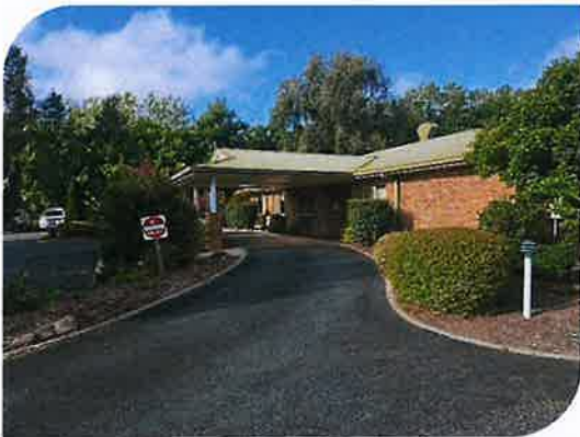
Figure 13 – The existing Administration Wing, looking south Source: K+C, 3 February 2026
