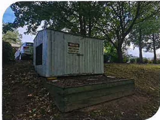
Figure 16 – Existing generator shed located to the south of the Site Source: K+C, 3 February 2026
