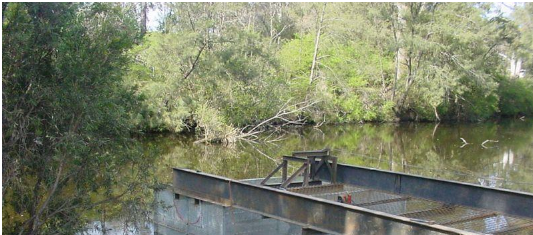
Figure 7-1 Tooloom Creek intake – UMMWWS Scheme
