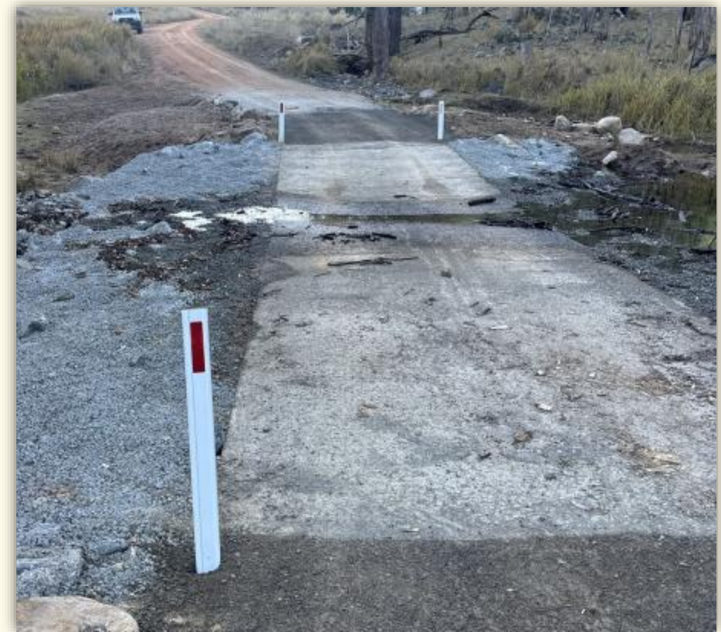
Eagle Creek Rd Causeway
