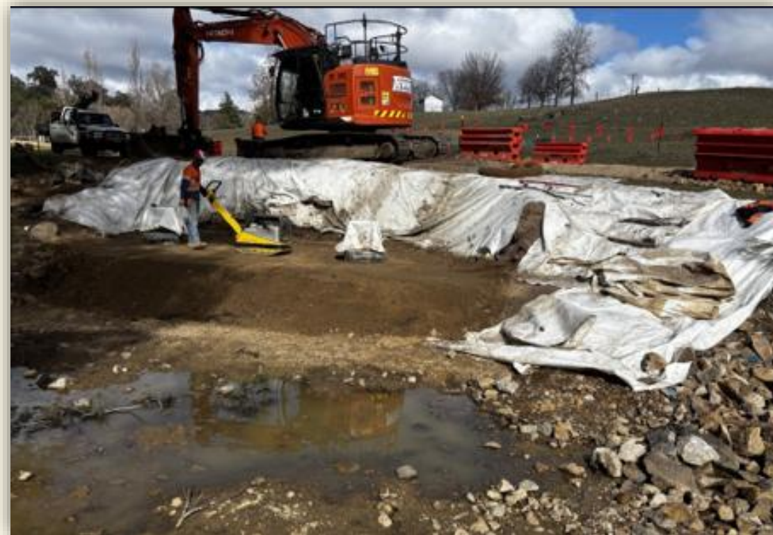
Bridge 2 scour protection
